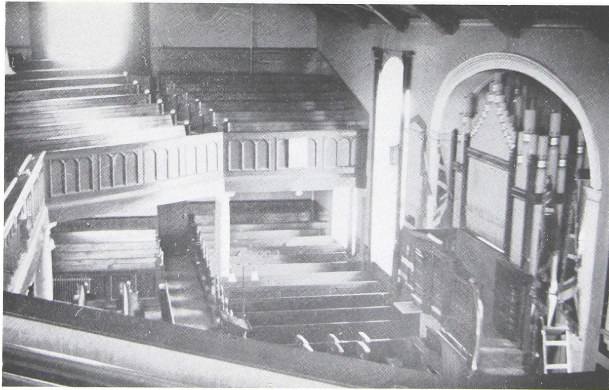
ELLON PARISH CHURCH: INTERIOR BEFORE RENOVATION
