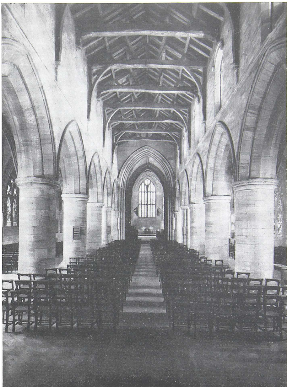
Nave – looking east
