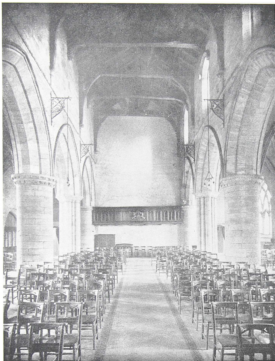
Nave – looking west, showing partition wall
