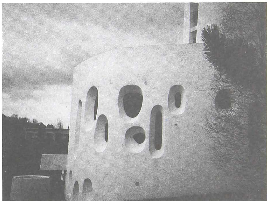
37 La Chaux-de-Fonds, Switzerland : St John's church
